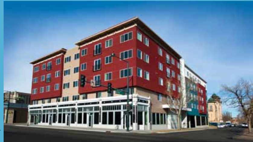
Renaissance Uptown Lofts in Denver opened in December, 2010.
